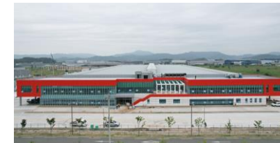
산업설비 (Industrial Facility)
